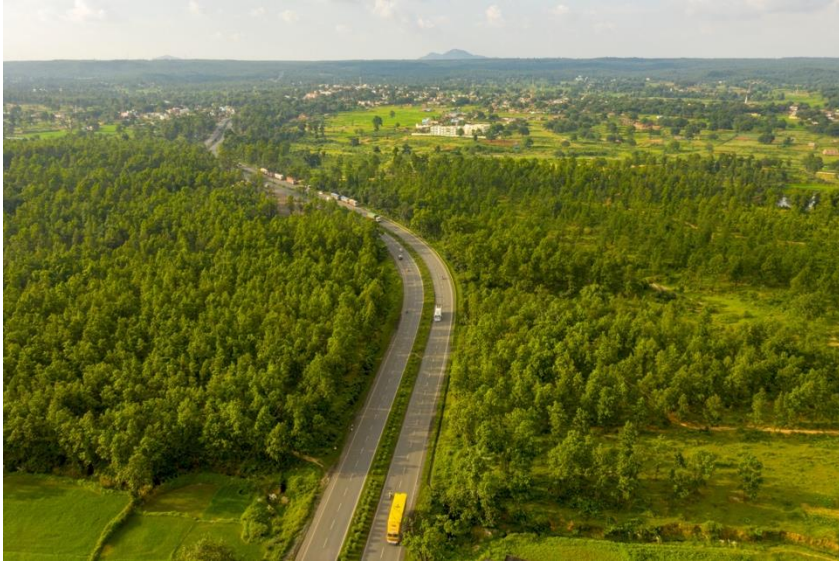
Barwa Adda Expressway Limited (BAEL)
