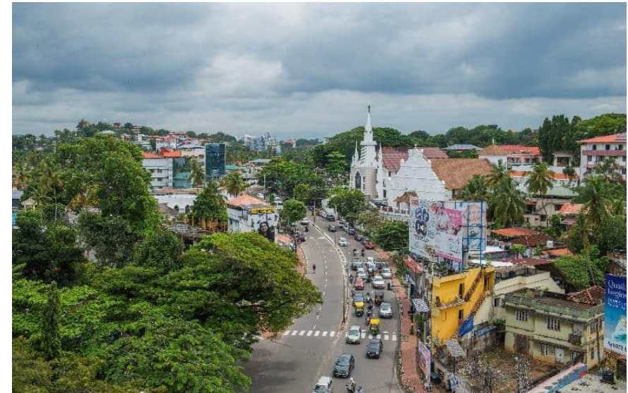
Thiruvananthapuram City Roads Improvement Project (TCRIP) in Kerala involved constructing, operating, and maintaining 10 corridors and 3 NH-bypass links totaling ~102.08 km
